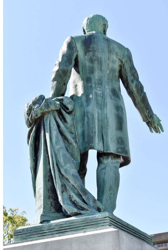
Fig. 4 - Back of figure. Heavy verdigris patina with uneven blotchy dark areas and carbon staining
