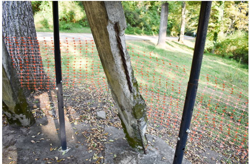
Fig. 11 - Large sections of loss on pillar exposing rebar sections. Shoring posts aiding in support
