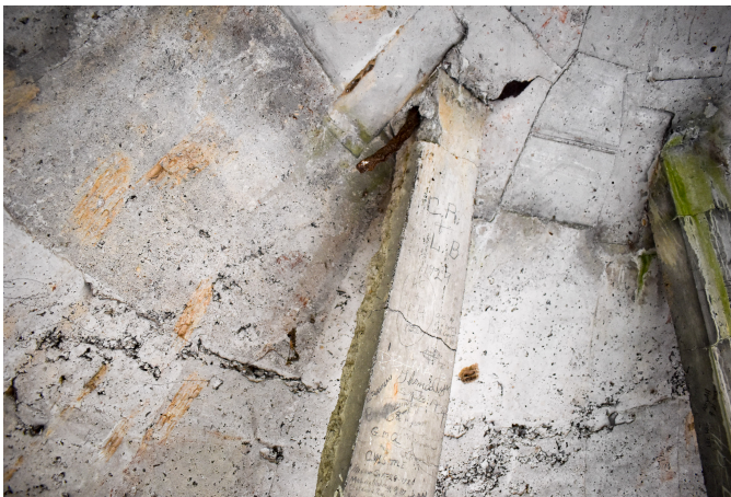
Fig. 5 - Detail of exposed rebar damage, historic graffiti on pillar, and fracture. Numerous air pockets from fabrication within concrete
