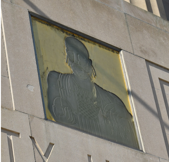
Fig. 5 - Justinian. Gold leaf deterioration along top edge.
