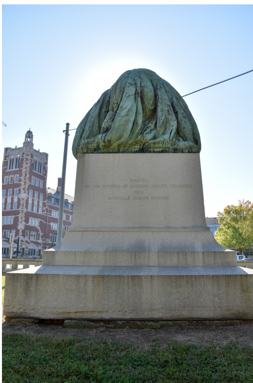
Fig. 3 - Overall vantage / back. Concrete footer exposed, abrasions visible on lower stone
