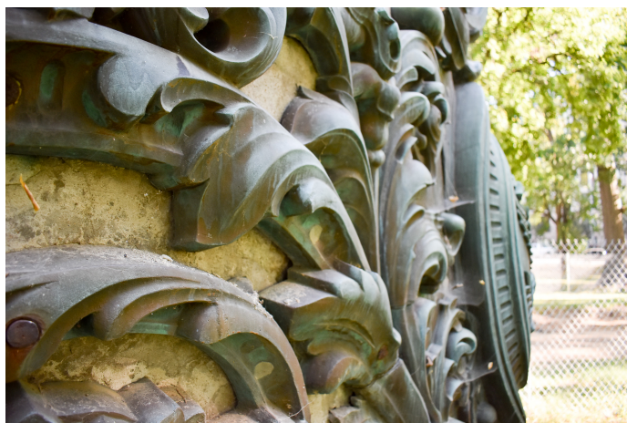
Fig. 5 - Detail showing corrosion staining from iron, light brown paint drips, debris and verdigris
