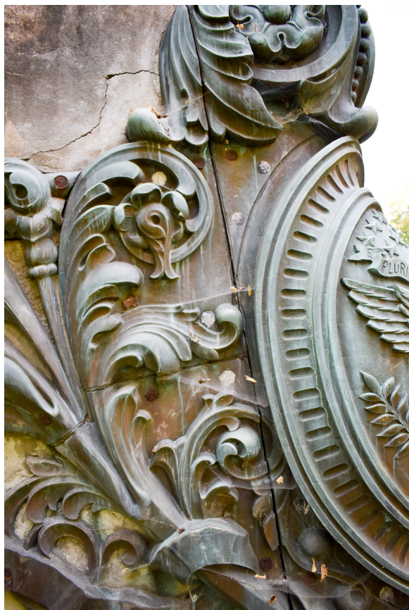
Fig. 6 - Detail showing corrosion staining from iron, light brown paint drips, and joining of sections
