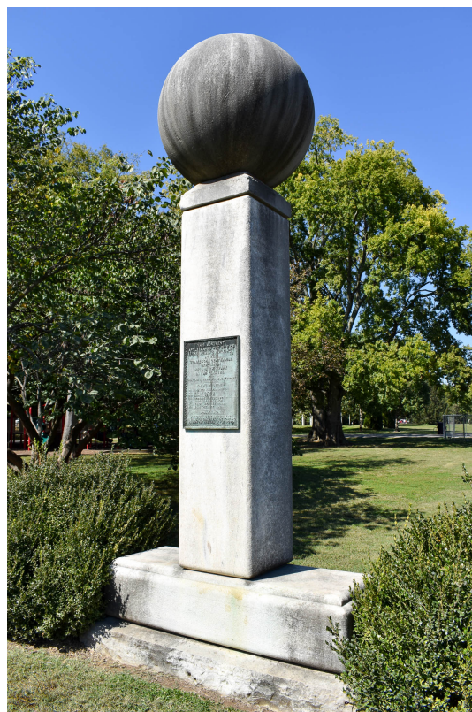
Fig. 3 - Biological staining, oxide runoff on lower portion of base
