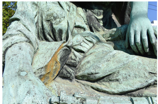
Fig. 10 - Verdigris corrosion and unidentified rust staining on satchel
