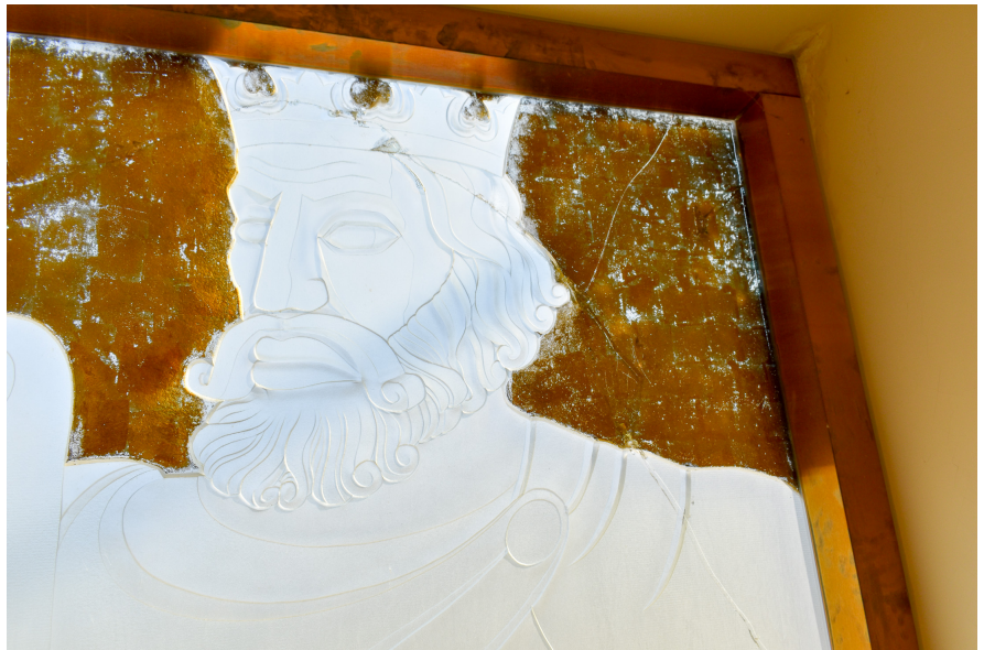
Fig. 11 - King John detail showing crack network, spalling in the crown area, gold leaf deterioration, oxidation on copper alloy, and water staining in drywall upper right corner. Further investigation is needed to find source of water ingress.
