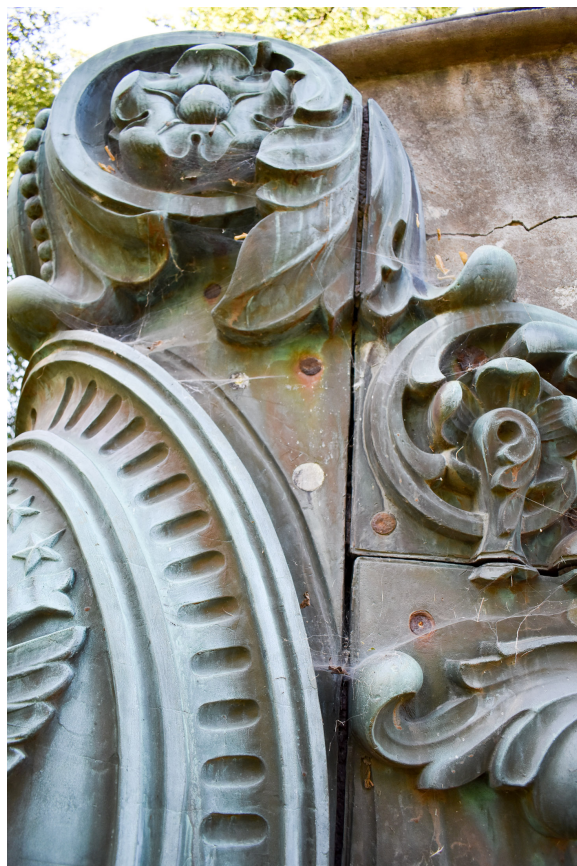
Fig. 7 - Detail showing corrosion staining from iron, light brown paint drips, and joining of sections
