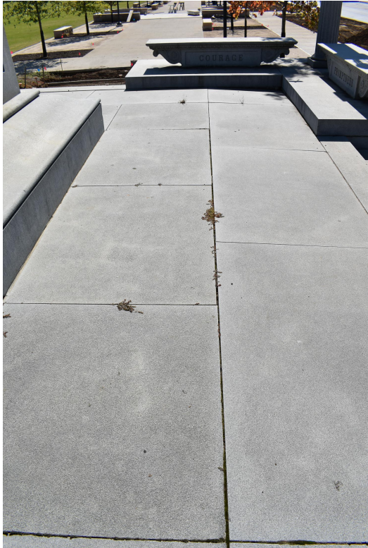
Fig. 12 + 13 Seam losses/plant growth in cavities throughout flooring
