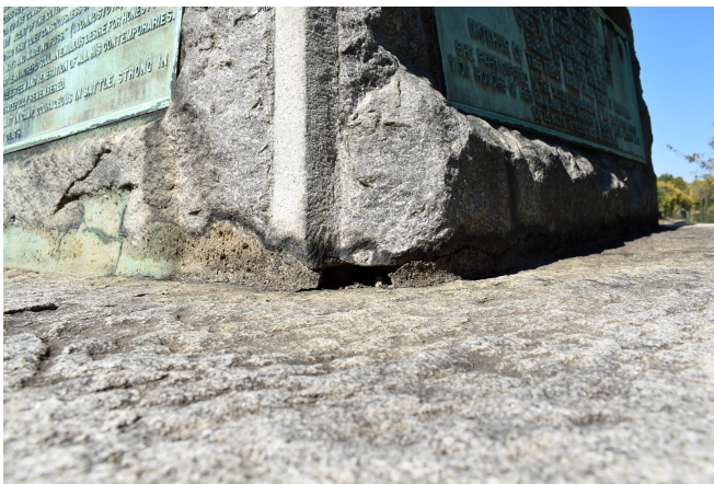
Fig. 7 - Mortar loss and staining
