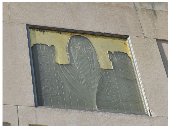
Fig. 4 - Moses. Large, curved crack from right shoulder to sternum - repaired. Gold leaf deterioration. Limestone loss on lower right corner
