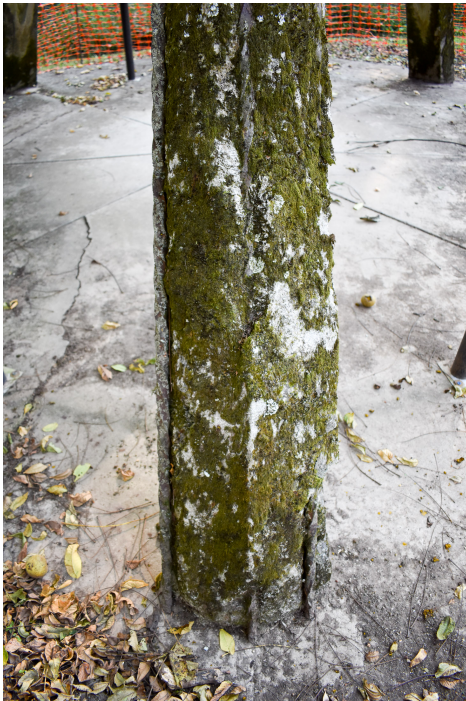
Fig. 10 - Lower pillar section. Exposed rebar, heavy biological growth.
