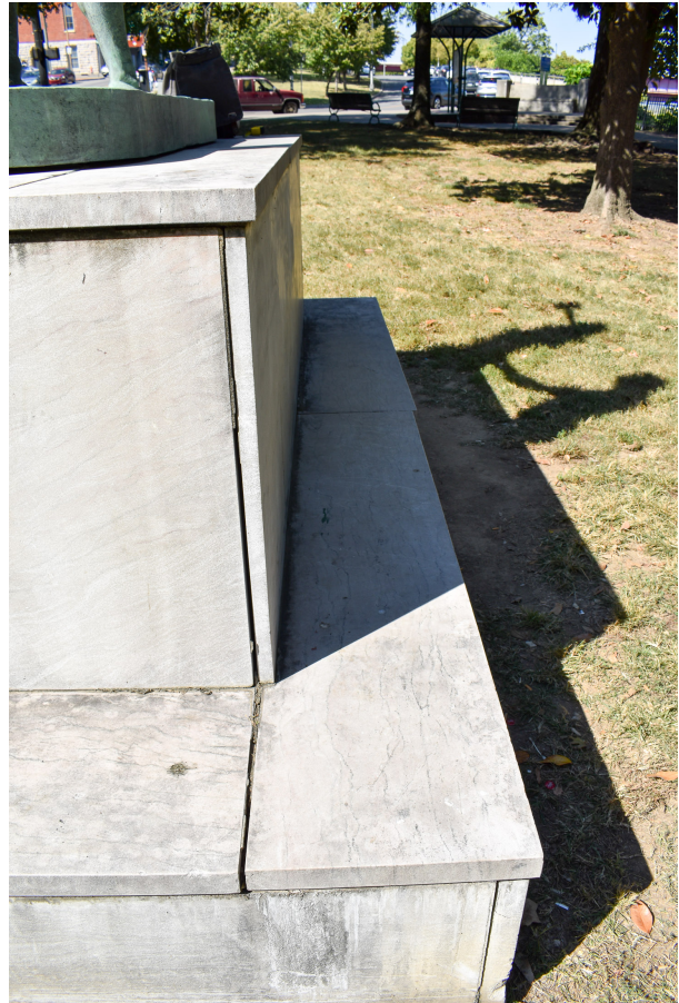
Fig. 8 - East face out of plane (lower tier). Bio staining on base, gouges from lawn mower, mortar losses
