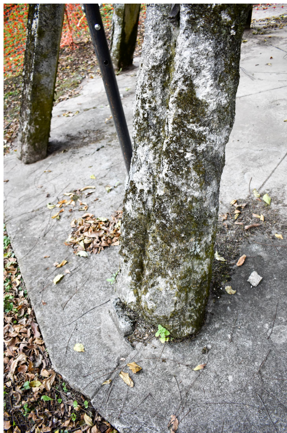
Fig. 2 - Heavy biological growth development and rebar segment loss (rebar intended to fit in channel slot)
