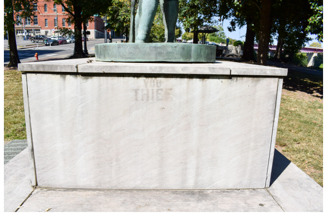
Fig. 6 - Mortar seam losses, staining, and ghost image of graffiti: "YOU THIEF"
