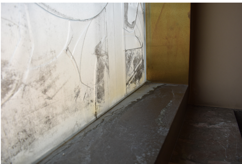
Fig. 14 - Detail of white liquid staining on copper alloy framing.
