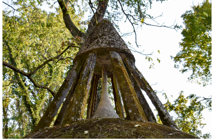
Fig. 9 - Upper cone section. Multiple areas of exposed rebar and partially intact pillar structures, fractures possibly hidden due to moss growth.
