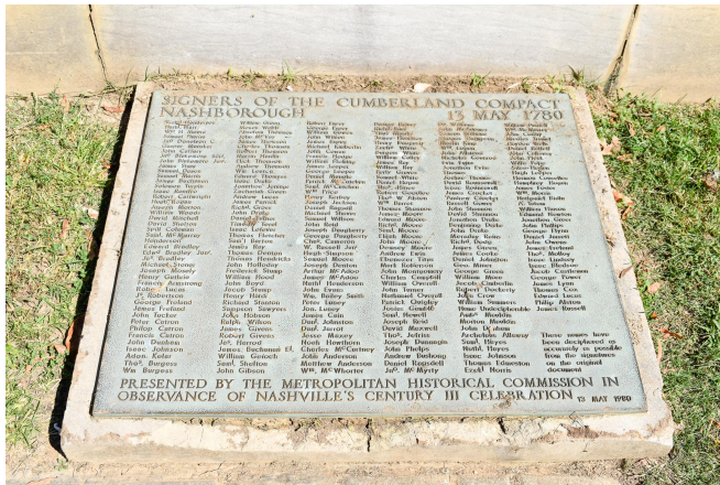
Fig. 1 - Ground plaque showing oxidation and concrete loss
