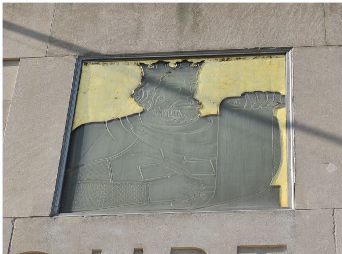
Fig. 3 - King John. Gold leaf deterioration along top edge.
