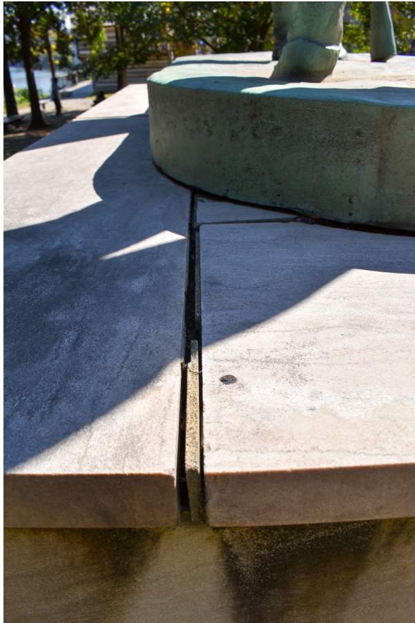
Fig. 7 - Typical losses and gaps in all seams between marble slabs
