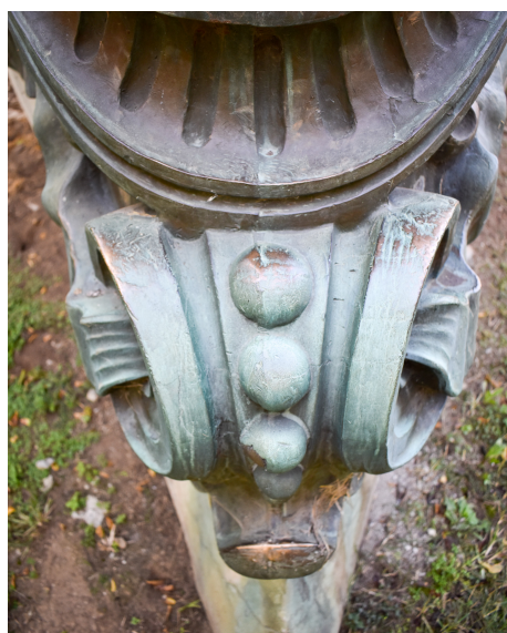
Fig. 8 - Detail from crest - worn patina from climbing
