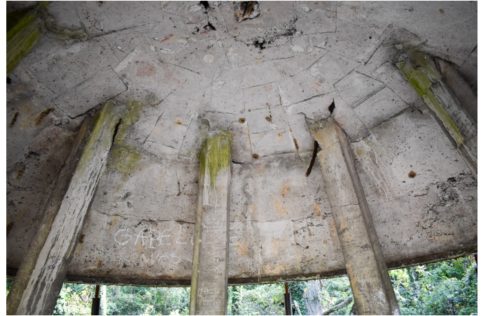
Fig. 4 - Dome underside opposite vantage. Rebar protruding through upper pillar. Losses, staining, and biological growth
