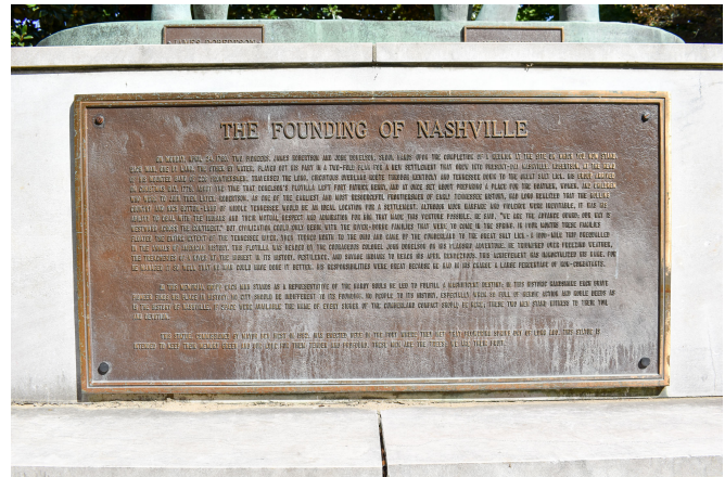
Fig. 2 - Plaque on sculpture base showing graffiti ghosting, failed lacquer.
