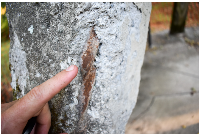
Fig. 7 - Detail to show scale of an exposed rebar section of pillar mid-point
