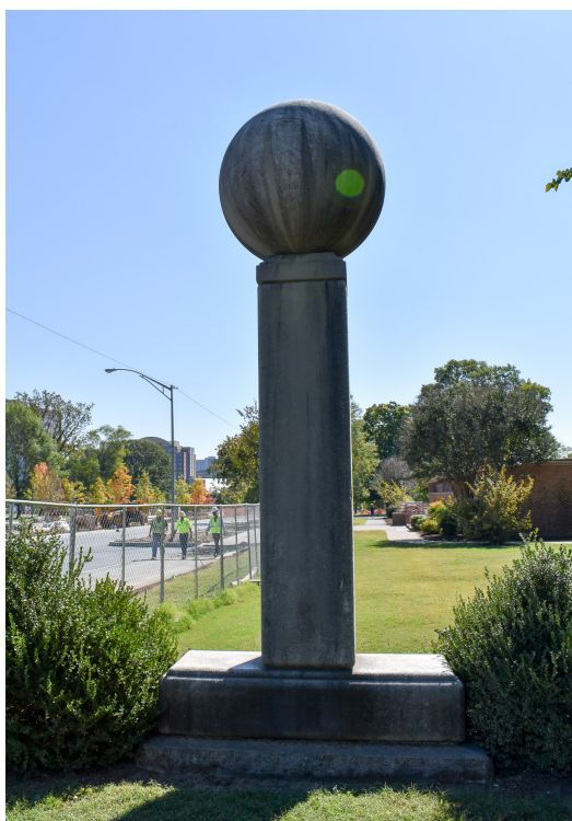
Fig. 4 - Biological staining on all surfaces
