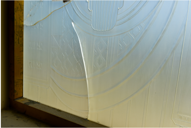
Fig. 8 - Moses interior showing larger fracture (see fig. 4 for exterior) Oxidation and staining on copper alloy framing
