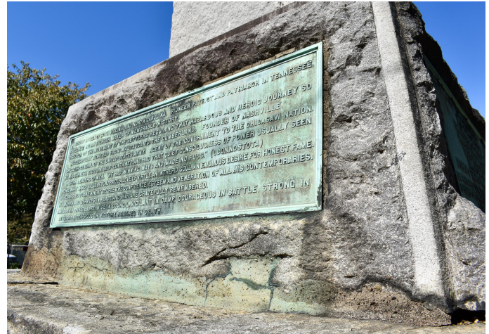
Fig. 6 - Plaque four showing verdigris runoff staining on mortar seams and fills
