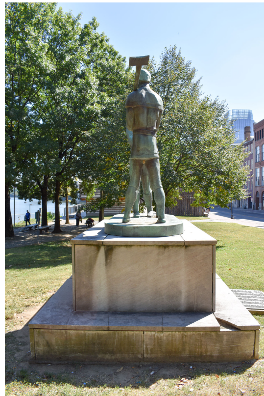
Fig. 4 - North vantage. Bio-staining on base, mortar losses, and verdigris corrosion on statues
