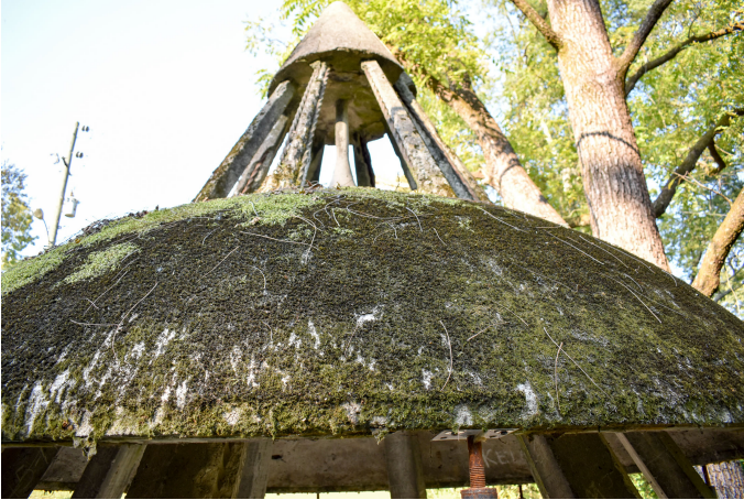
Fig. 8 - Heavy moss and lichen growth on outer dome. Exposed rebar sections on upper pillars.
