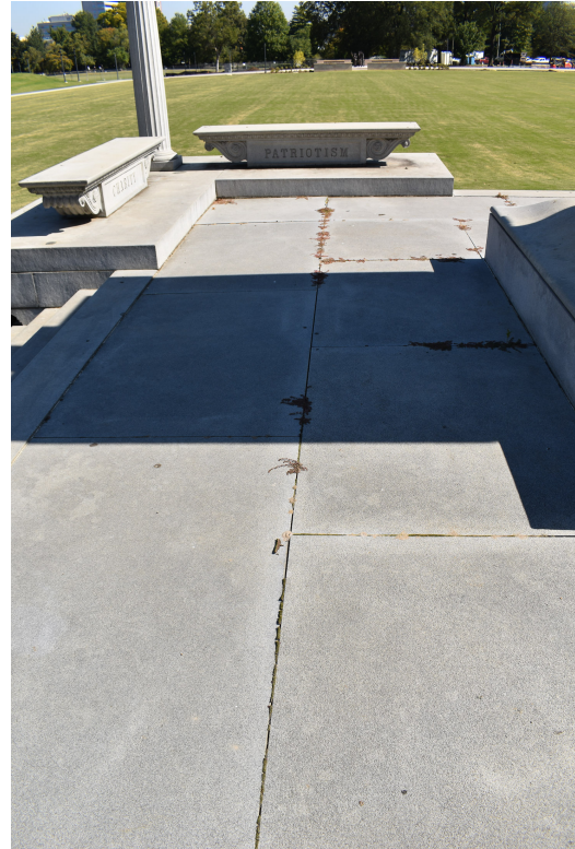
Fig. 12 + 13 Seam losses/plant growth in cavities throughout flooring
