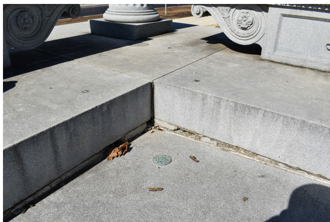
Fig. 10 - Concrete losses at corner
