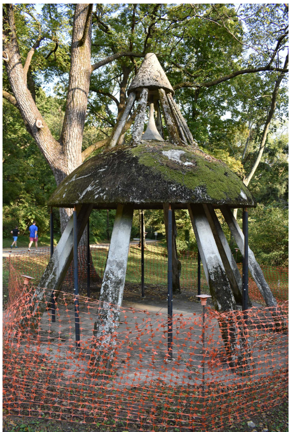
Fig. 1 - Overall vantage showing heavy moss and lichen growth on dome. Shoring posts aiding in structural support
