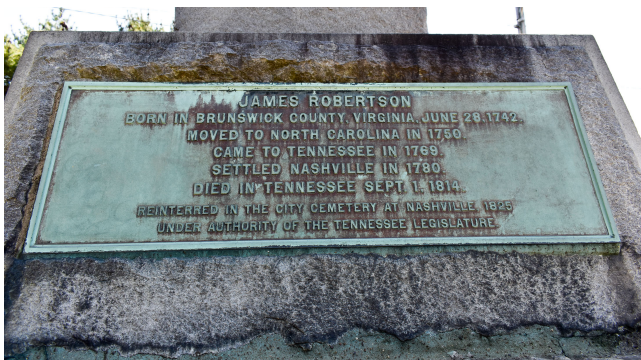
Fig. 3 - Plaque one with verdigris staining
