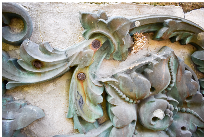
Fig. 4 - Detail showing corrosion staining from iron, light brown paint drips. Wasp nest
