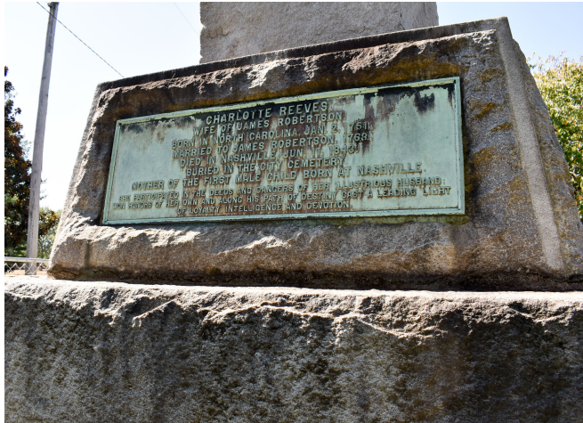
Fig. 5 - Plaque three showing verdigris and carbon crust. Bio staining on base
