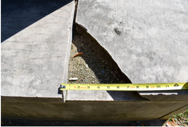
Fig. 5 - Extent of large loss on base
