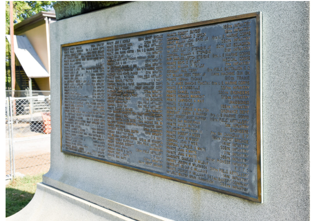
Fig. 6 - Plaque / left side showing failed lacquer.
