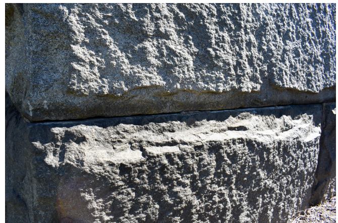
Fig. 8 - Mortar pointing loss (2' L section)
