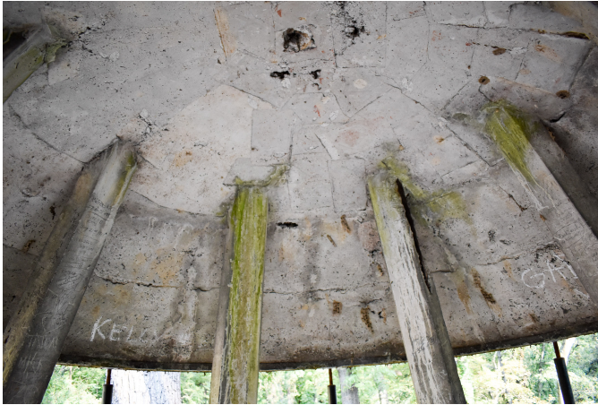
Fig. 3 - View of dome underside showing losses, exposed rebar and graffiti
